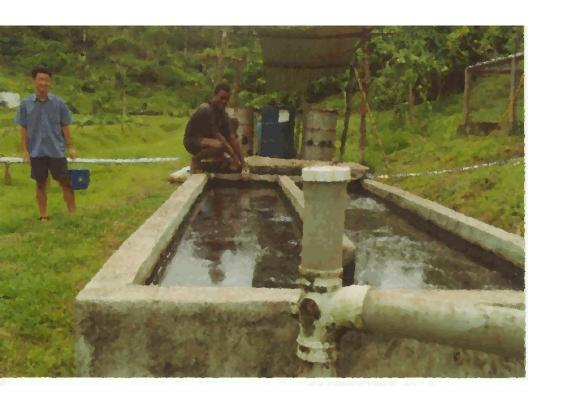
Sedimentation tanks can be built with numerous easily accessible materials.
